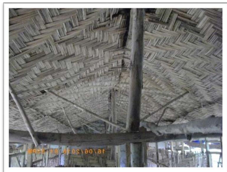
Fig. 3 picture of Local Talamat as insulation
